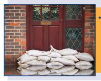
Build a small sandbag wall across external doorways. This includes sliding doors and garage roller doors. The height of the sandbag wall will depend on the expected height of the floodwater; however, it is generally around two sandbag rows high.
