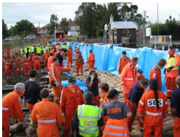
ACTSES teams assist to build a sandbag wall against floodgates in preparation for the flood peak. Photo: Rebecca Noble.
